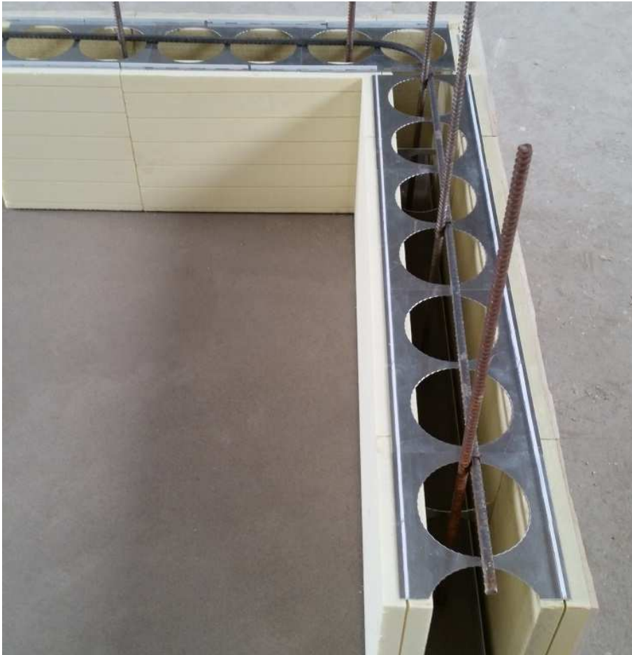
Set horizontal re-bar and tie to vertical starter bars
