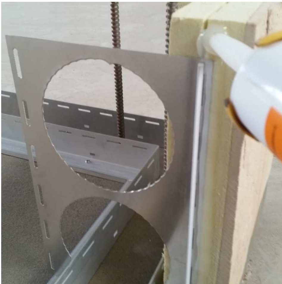
Apply sealant along and adjacent to joiner
