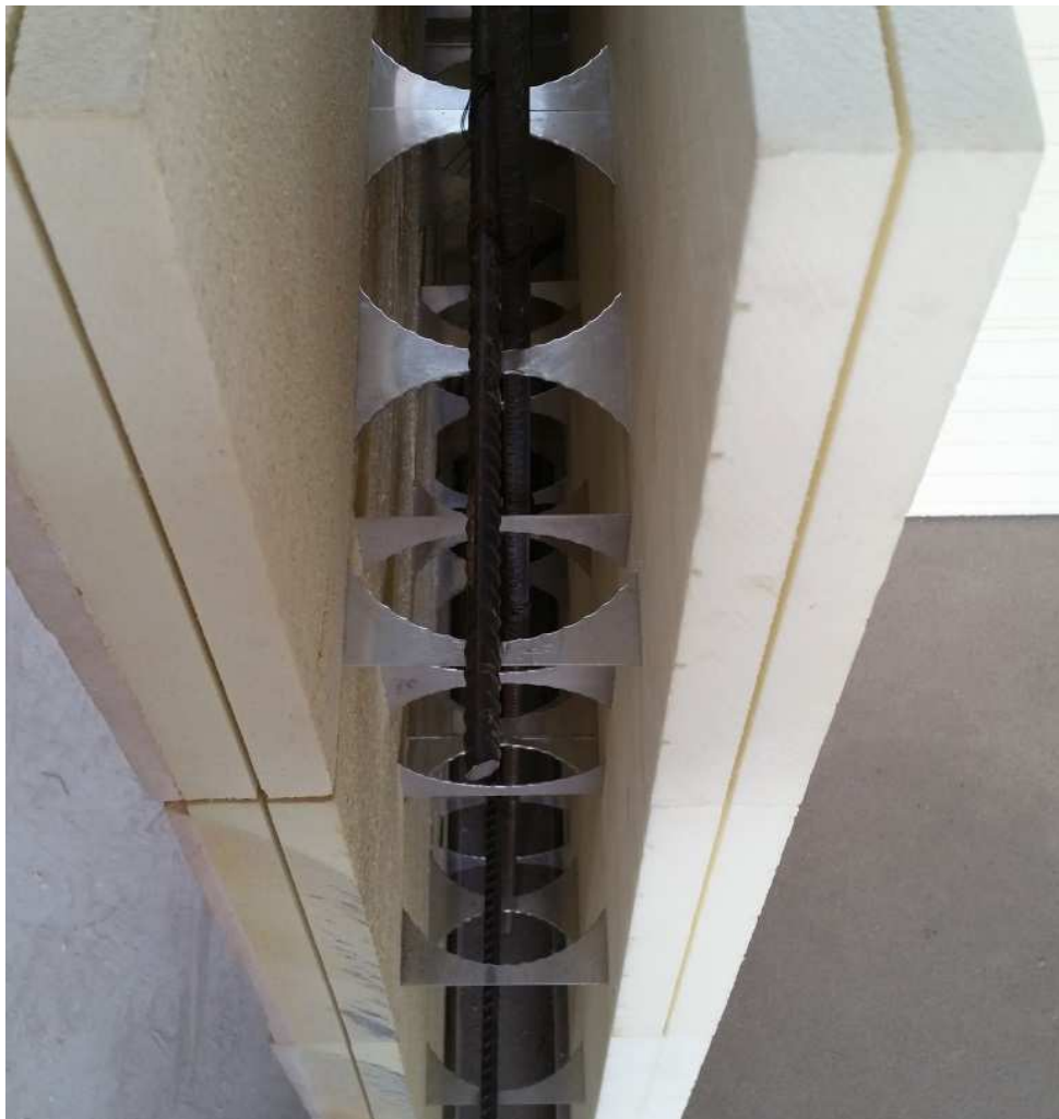
The cavity before closing up for concrete pour.
