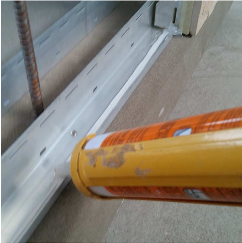
Apply sealant to the bottom rail.
