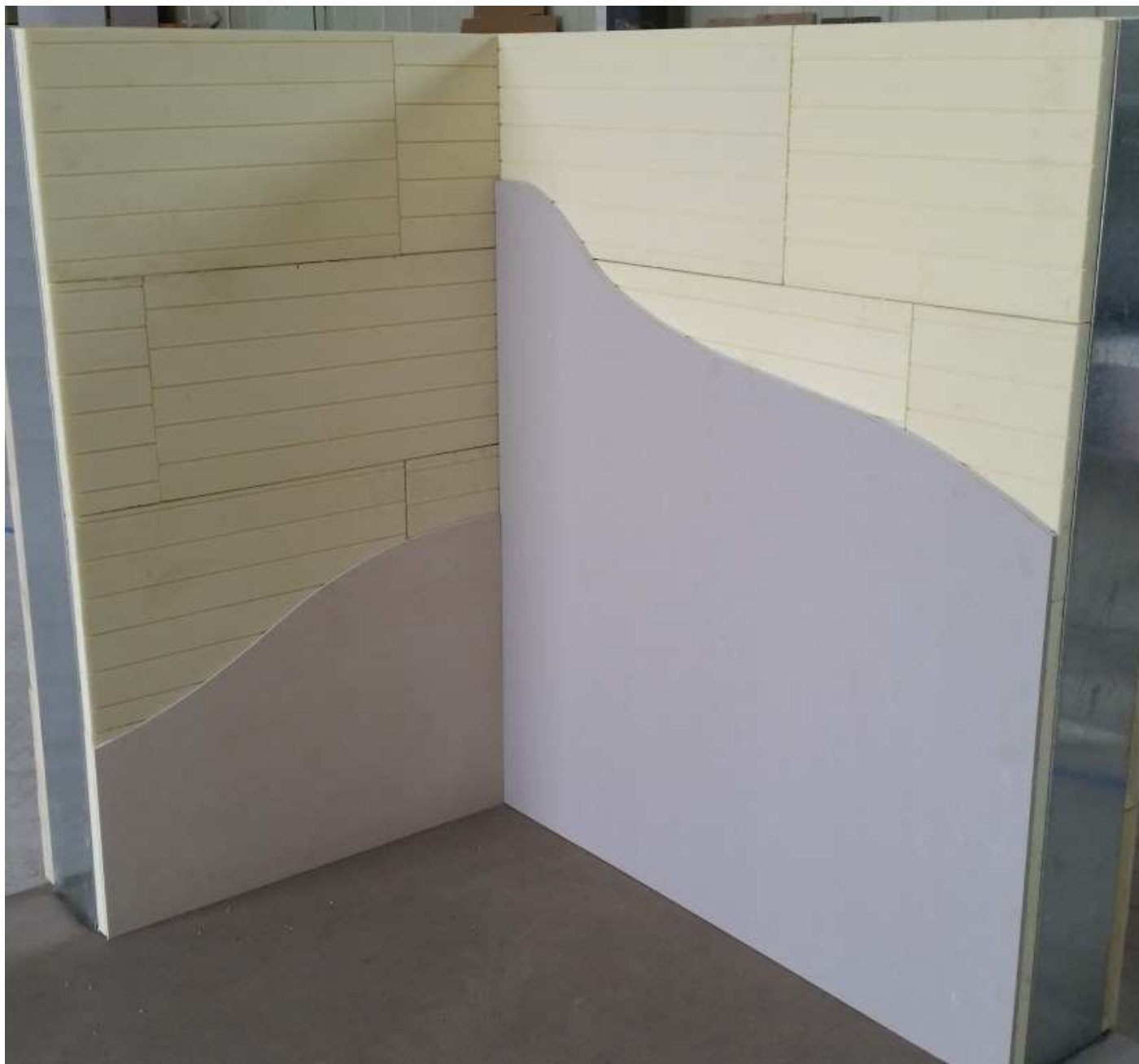
Internal walls simply drywall, right, for paint or ceramic tile directly over as on left.
