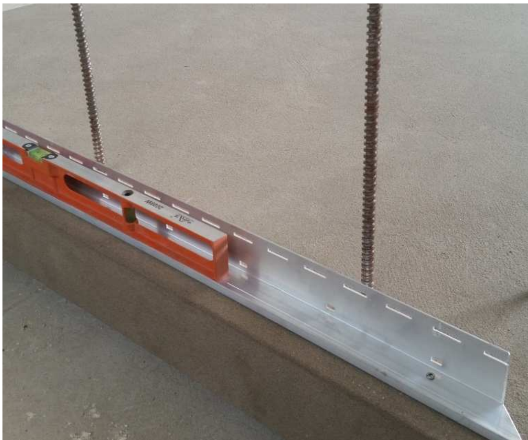
Outer starter rail set level and plumb, screwed and glued into place.
