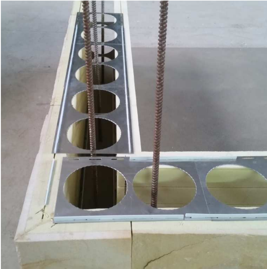
The brackets can all be set in place with the alignment joiners
