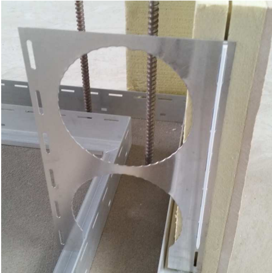
Place bracket into end groove aligned with PVC joiner
