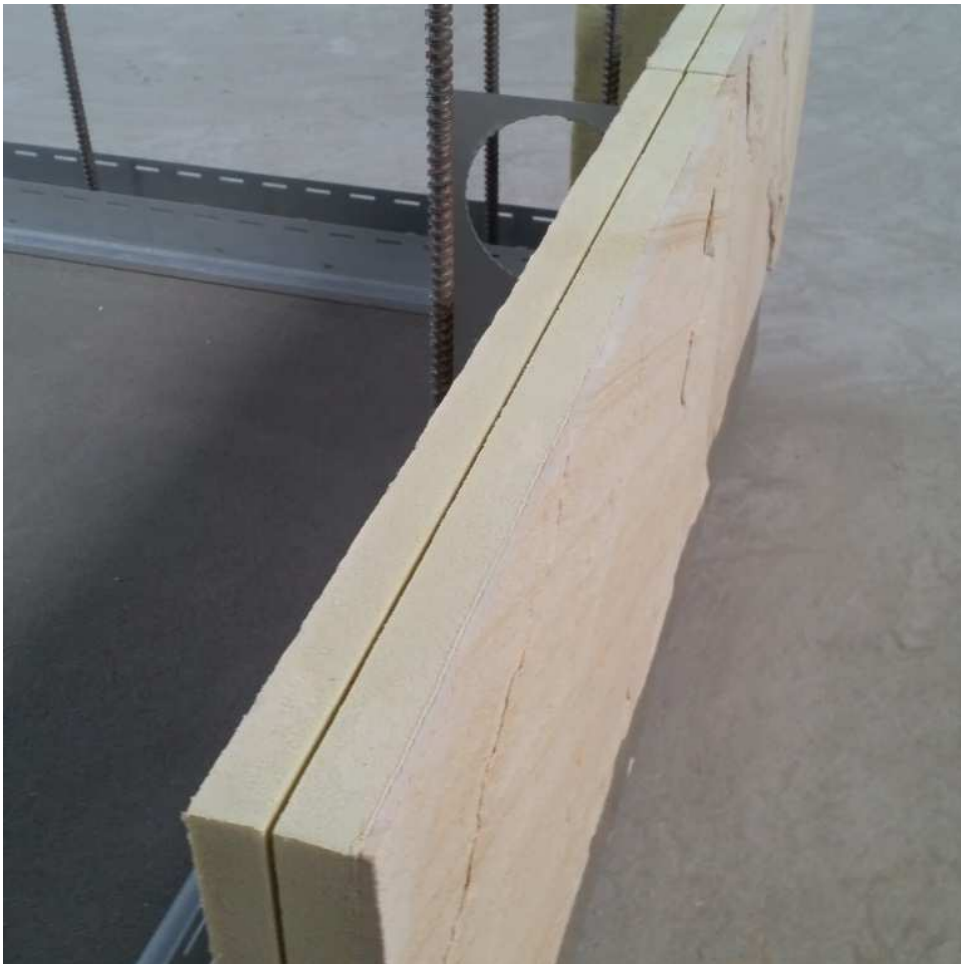
Position the next stone into place onto alignment grooves.
