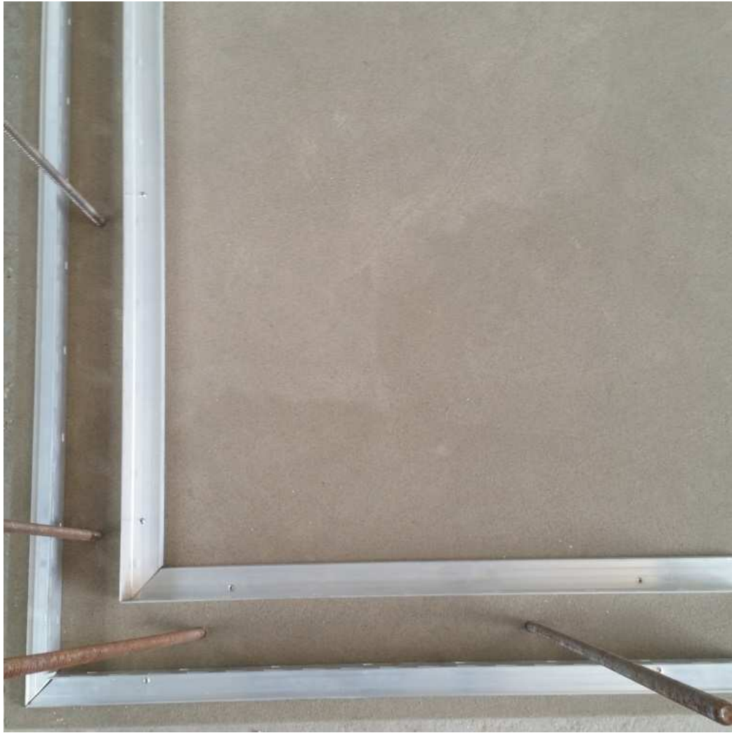
Internal rails fixed squarely and level
